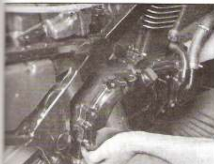
5.19 With the engine supported by a floor jack, have an assistant help you lower it and guide it out of the frame
