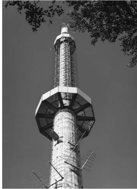
FIGURE 29-19 Typical broadcast antenna installations on a concrete supporting structure. A UHF TV antenna is mounted on top of the tower. It is protected by a GRP radome that is provided with helical strakes to reduce its vulnerability to mechanical oscillation at certain wind speeds. Below this is a VHF FM radio antenna built from dipole panels, and below this is a variety of LPDAs. (Courtesy of Kathrein-Werke KG)
